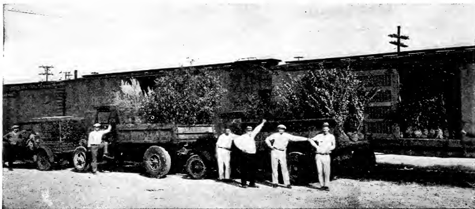
Unloading Shipment Containing 18 Truck Loads, at West Palm Beach for Repairing Storm Damage in That Section, Nov., 1928.
